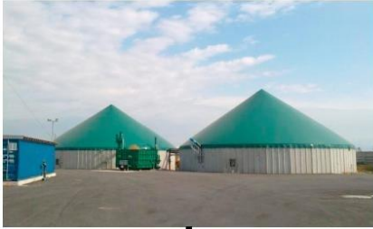
Anaerobic Digestion Plant
